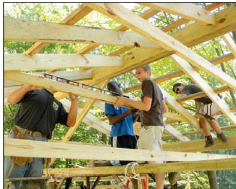
Teens help build an “access friendly” campsite at Kingswood.
