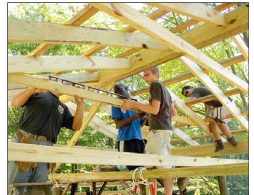
Teens help build an “access friendly” campsite at Kingswood.
