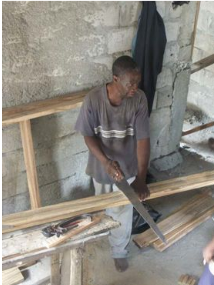
Carpenter at work on the Parsonage/Conference Center
