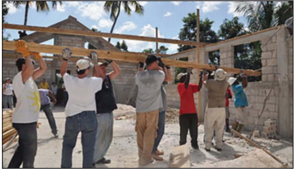
The team helps hoists a beam in place to support the rafters.
