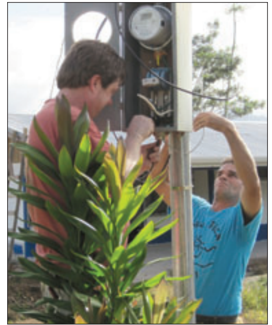
ABOVE: Philip Koerner and Juan work to wire an electrical panel outside the school. LEFT: The volunteers begin preparations to finish off a classroom ceiling.
