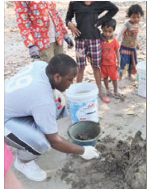
Christopher Blair, left, mixes cement that will be used to secure fence posts in the ground.
