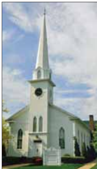
The steeple of First Church has been a beacon of faith in Baldwin.
