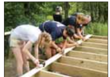
Participants in the Woodsmoke program work on the tent platform, above, and pour concrete for the platform footings, at left.
