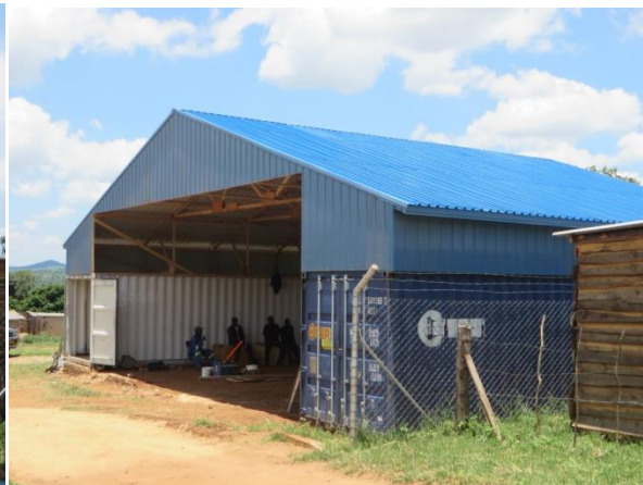
The VIMs (along with the locals) built tractor and farm equipment shed using the two containers as the feet of the roof. The shed is to protect the tractors and farm the equipments from the effects of harsh weather. We shall talk more and show more pictures on the various activities of the VIM team in the next newsletter. Don't miss it.
