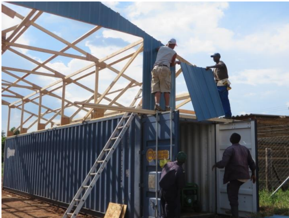
The VIMs (along with the locals) built tractor and farm equipment shed using the two containers as the feet of the roof. The shed is to protect the tractors and farm the equipments from the effects of harsh weather. We shall talk more and show more pictures on the various activities of the VIM team in the next newsletter. Don't miss it.
