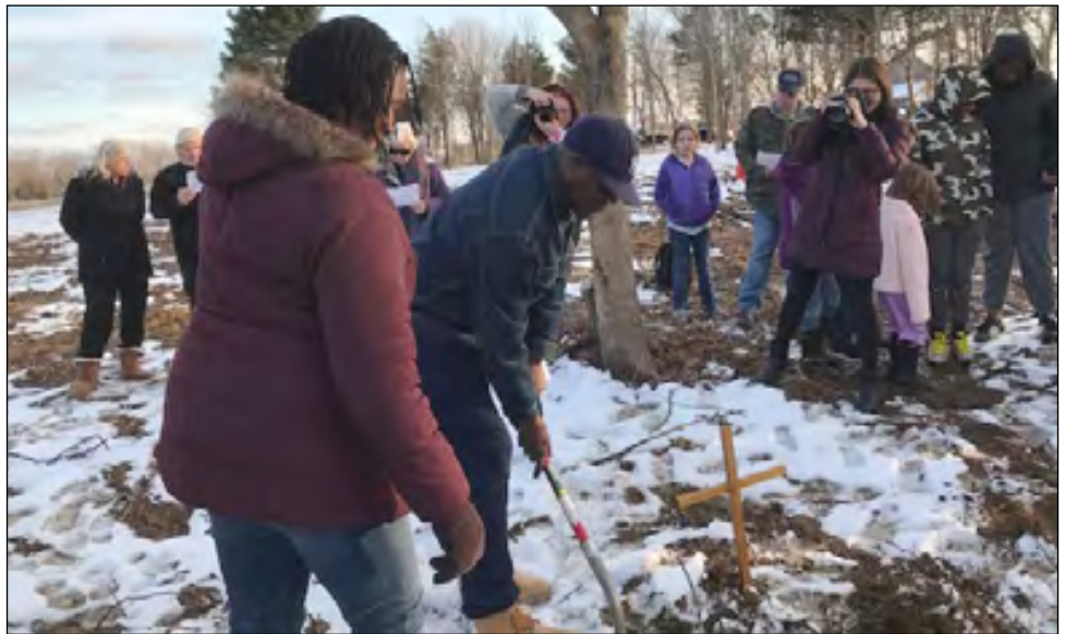
Members of the North Fork, above, UMC break ground around a small cross for their new church building in Southold, N.Y. Below, Pastor Tom MacLeod and District Superintendent Julia Yeon-Hee Yim, stand ready with a shovel before the ceremony.
