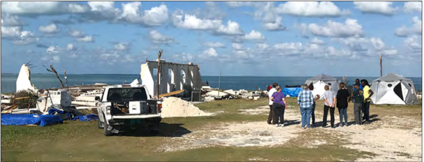
The chapel at St. Paul's Methodist Church in Freeport sustained significant damage.
