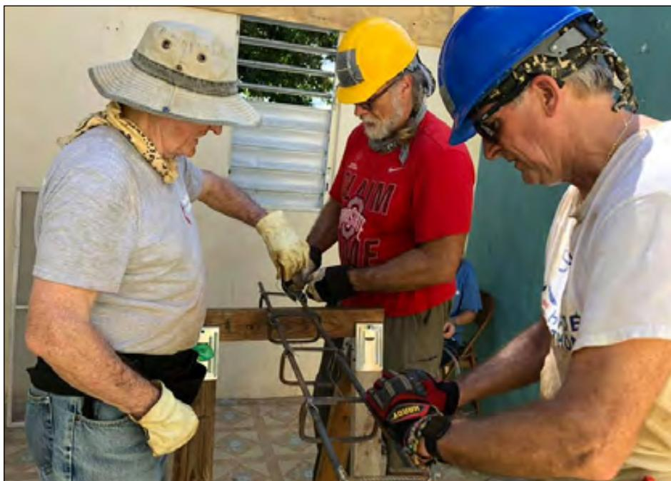
Rebar is cut and tied, above, to reinforce the exterior walls being constructed by an NYAC mission team, below, at a home in Puerto Pico
