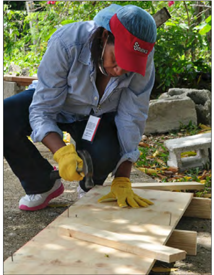
Building a frame for concrete foundation.
