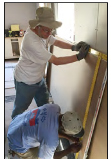
Tim Riss, top, and Joseph Ewoodzie team up to cut drywall.
