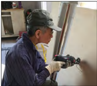
Sungchan Kim cuts an outlet hole in drywall.
