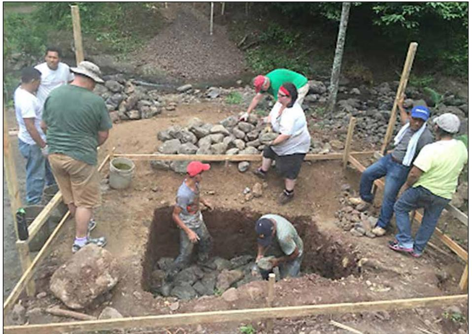
**Large rocks are placed in a hole before the cement that will form the footing on one side of the footbridge.**
